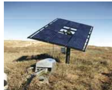
Solar Pumps Up to 5.8m 3 /h, 12 bar
